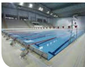
Indoor Sports Facilities
