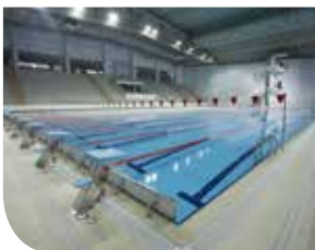
Indoor Sports Facilities
